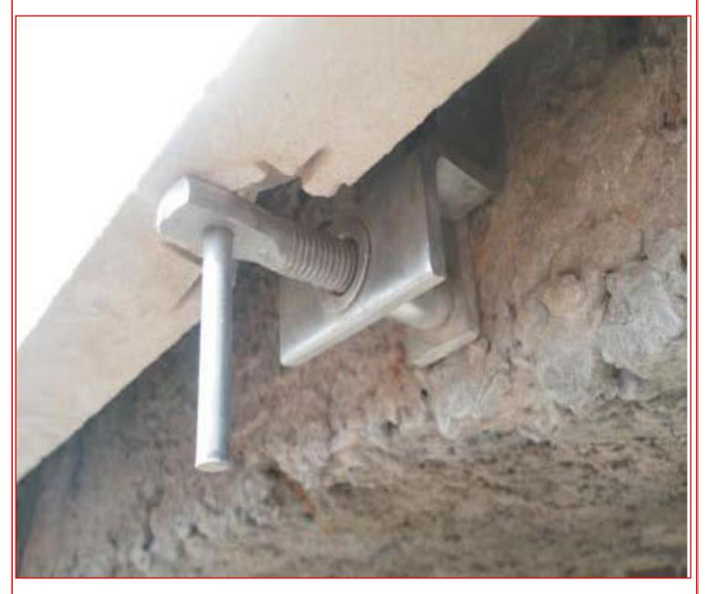
Fixing Solution For Natural Stone Cladding
